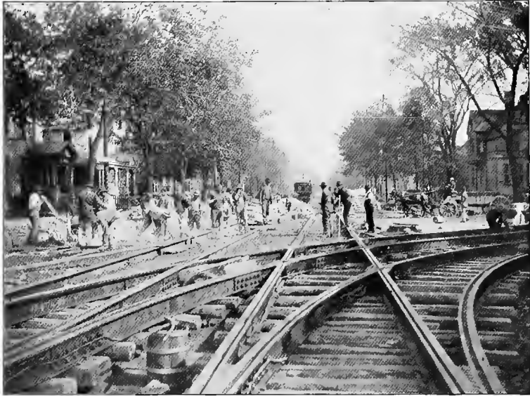
TRACK AND PAVEMENT CONSTRUCTION, ROCHESTER, N. Y., 1900.
